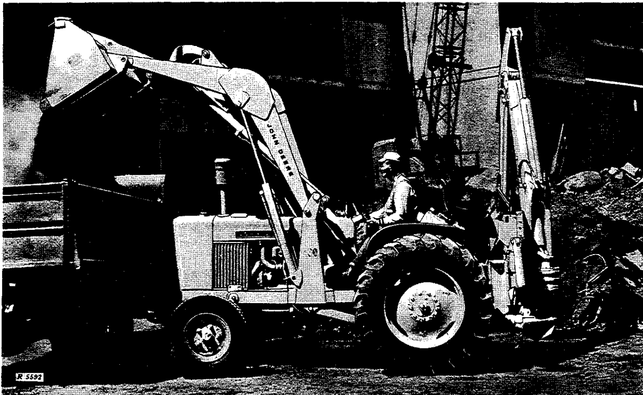
John Deere 3010 Wheel Tractor with Loader and Backhoe
